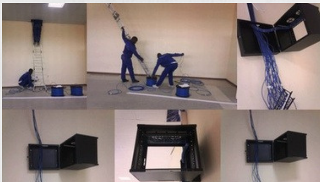
BAL PSI Network installation
